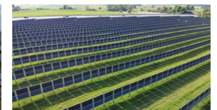
4.2MW Germany, 2020 Next2Sun Aasen PV Plant
