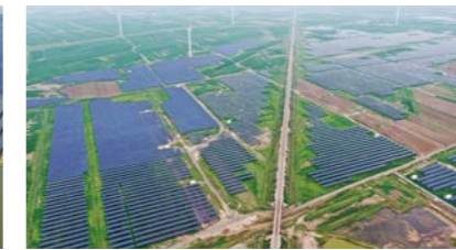
65MW Hebei, China, 2018 Haixing Top Runner Project
