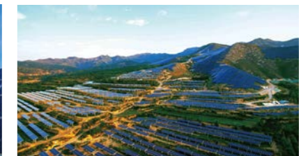
100MW Shanxi, China, 2017 Yangquan Top Runner Project
