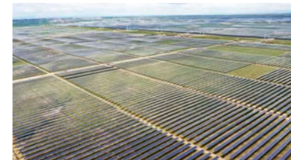
253MW Qinghai, China, 2020 Qinghai UHV PV Plant 2#
