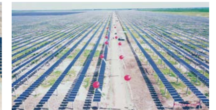
95MW Jilin, China, 2020 Jilin Baicheng Top Runner PV Plant
