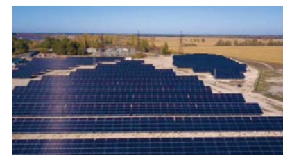
4.2MW Ukraine, 2019 Altes Chernobyl III PV Plant
